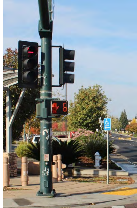
Pedestrian Countdown Signal Head
